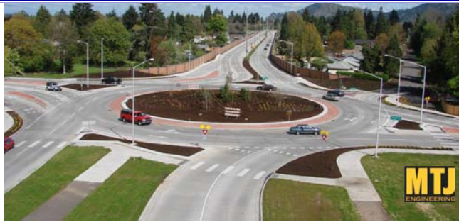
Springfield, OR: State of Oregon's First Urban Multi-Lane Roundabout (5,700 VPH Design Year Flow)
